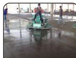
TPARK Warehouse (Bang Pli)
