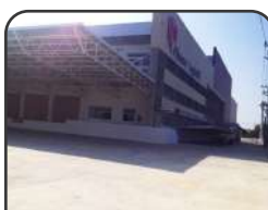
WHA Warehouse 4, 8, 9 (Bang Na)
