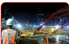
MRT Project PHOTO: JAYAMIX BY SCG
